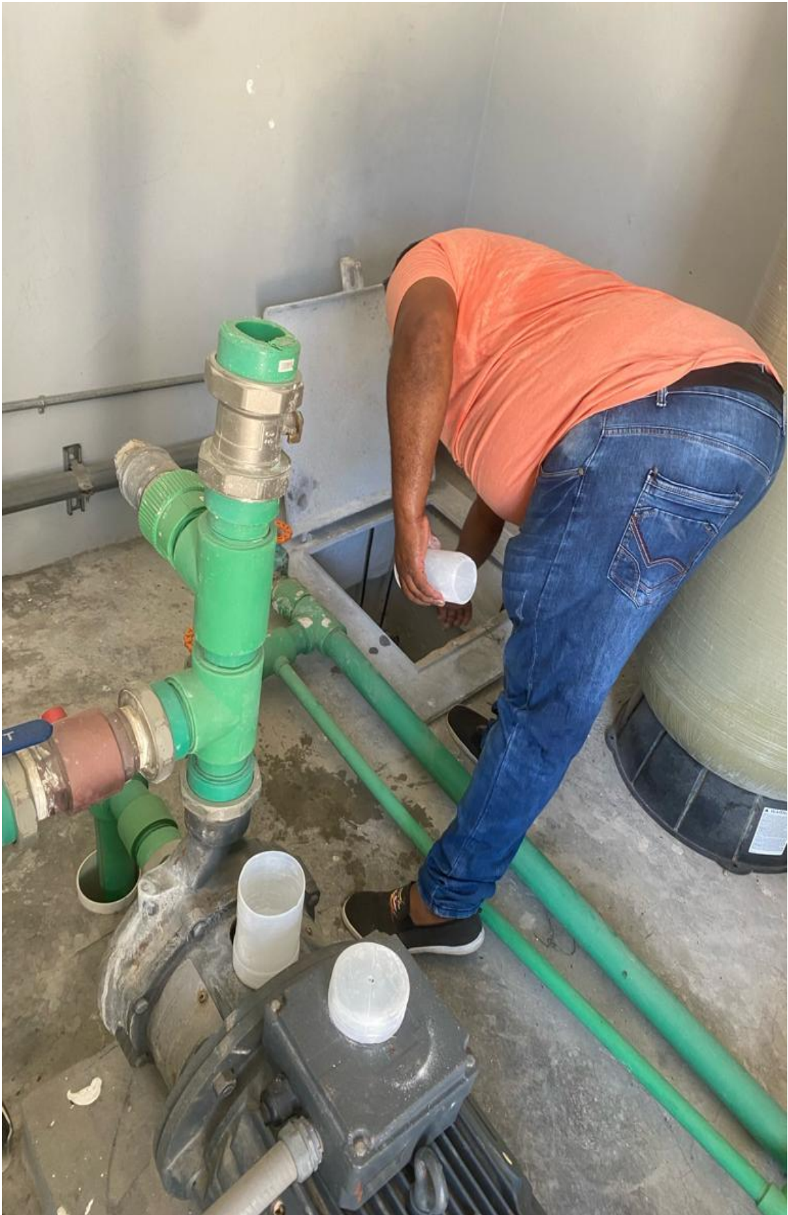
Clorificacion a cisterna 05/01/2024
