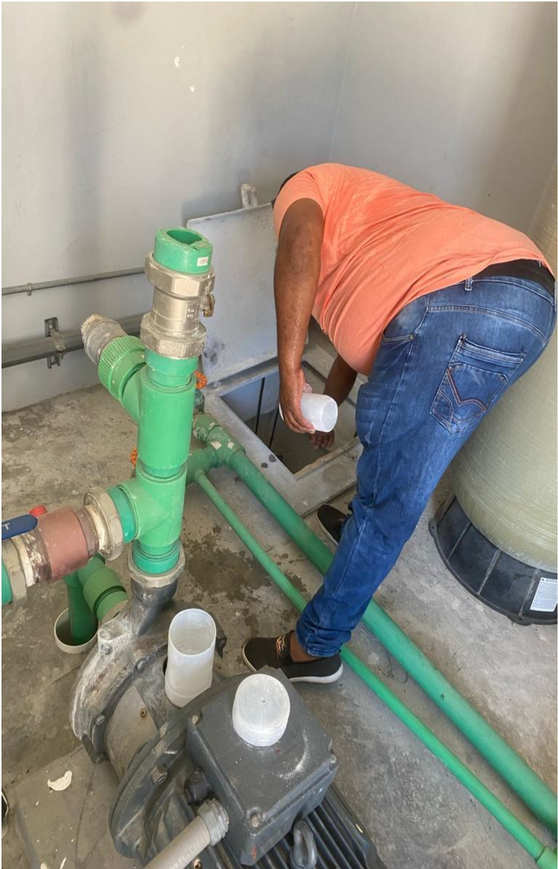
Clorificacion a cisterna 05/01/2024
