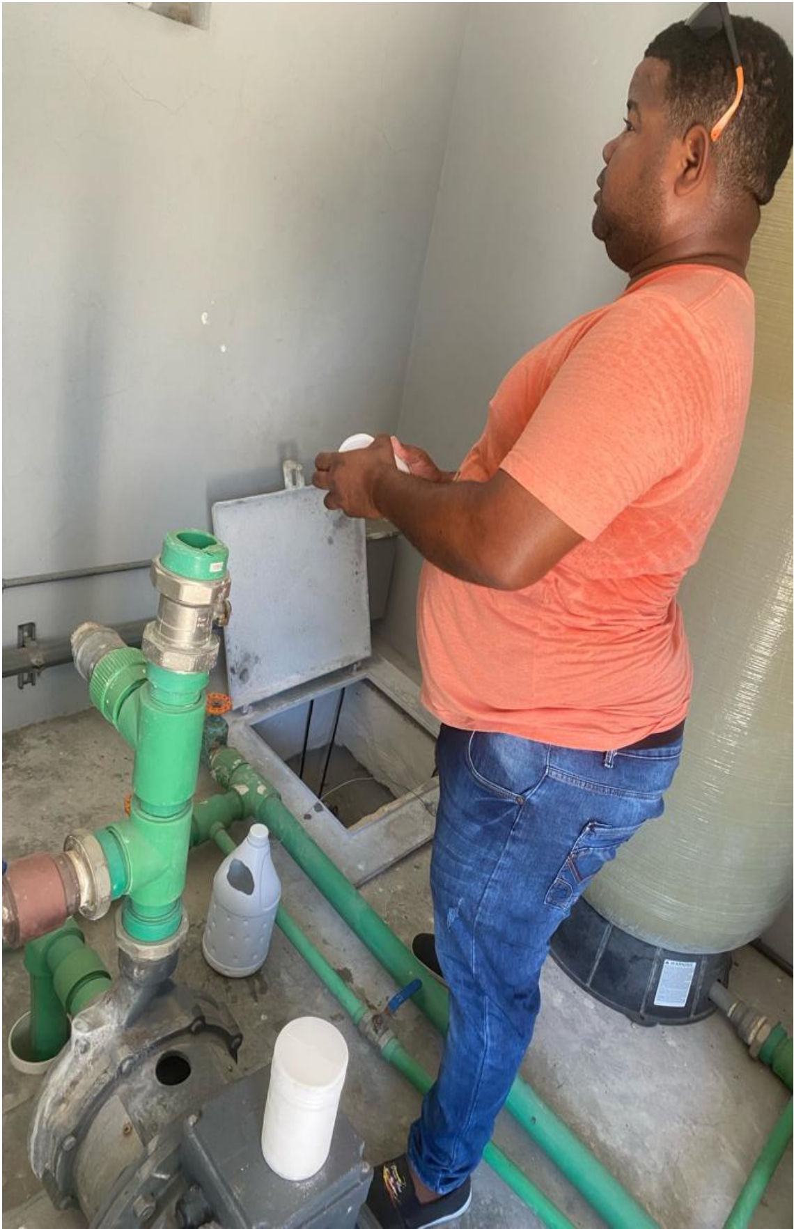
Clorificasion a cisterna 05/01/2024
