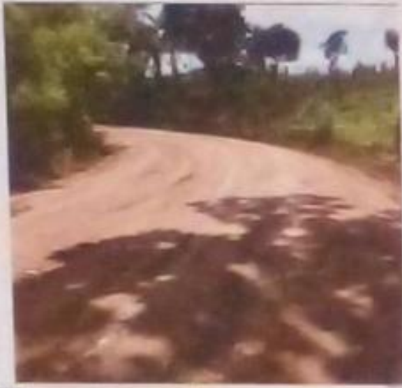
Carretera Bayaguana-Mata Santiago
